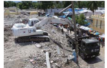
The Danbi Unit performing restoration work (June 2010)
