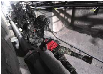
Inspection of underground conduit protection (May 2010)
