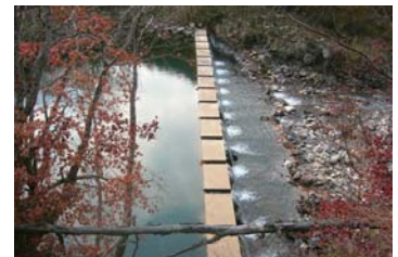
Regulating Reservoir Dam
