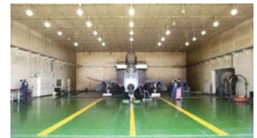
Inside View of a Soundproof Maintenance Shop
